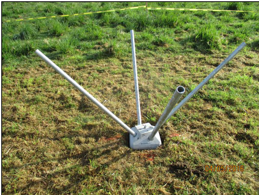
PHOTO 3: Typical concrete pier seated and ready for bearing pin installation.
