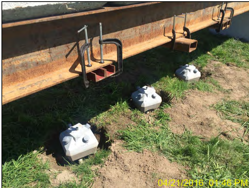
PHOTO 10: Diamond Pier DP-50 group load test alignment.
