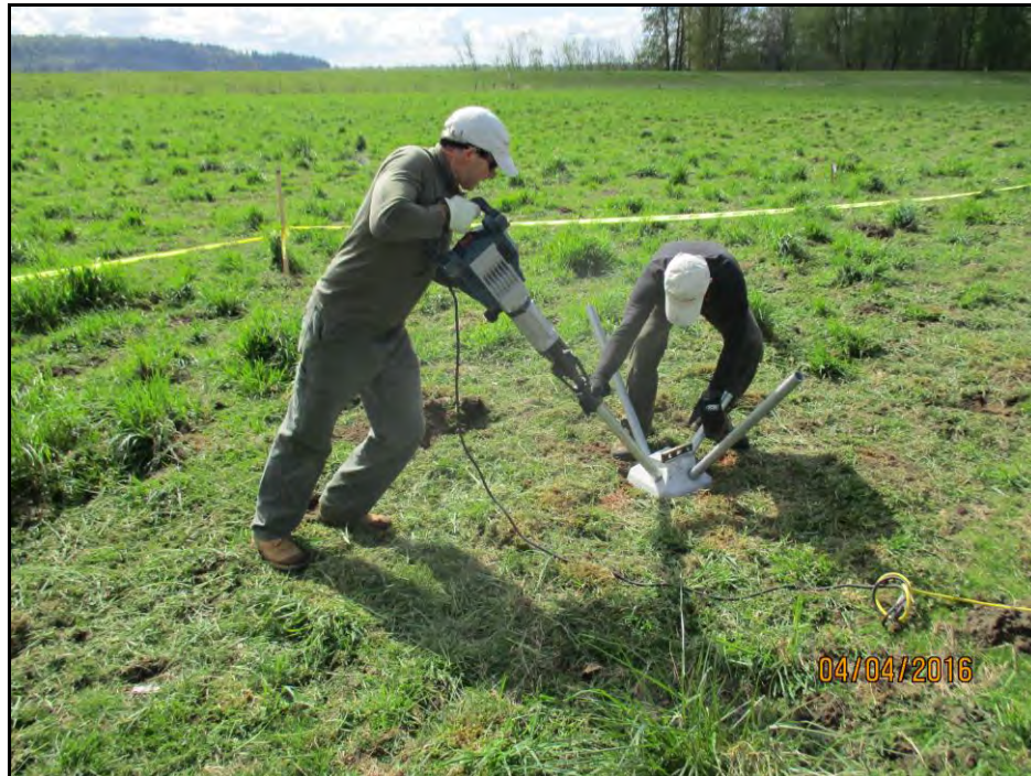
PHOTO 4: Typical driving of the steel bearing pins.
