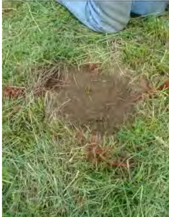
PHOTO 2: Sod removed in conical shape of concrete pier.
