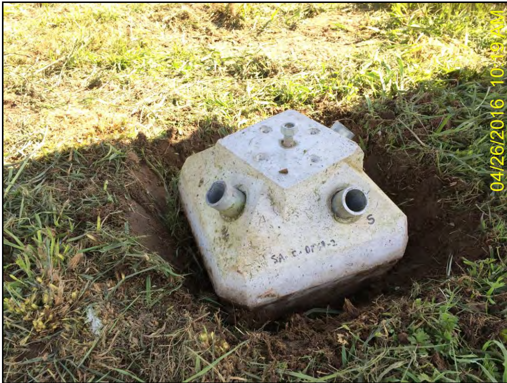
PHOTO 6: Typical Diamond Pier after 1 to 2 inches of soil were removed from around the bottom and sides.
