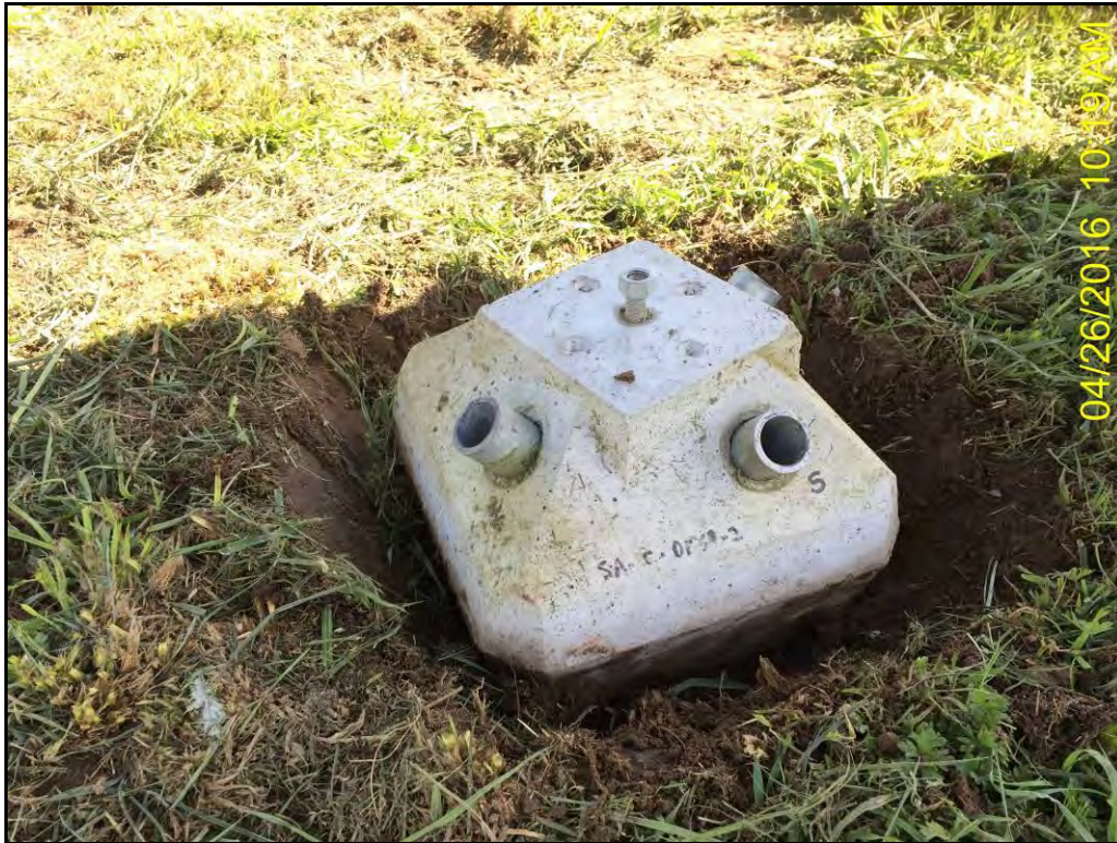
PHOTO 6: Typical Diamond Pier after 1 to 2 inches of soil was removed from around the bottom and sides.
