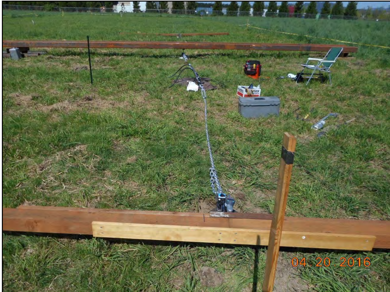
PHOTO 10: Typical lateral load test setup.
