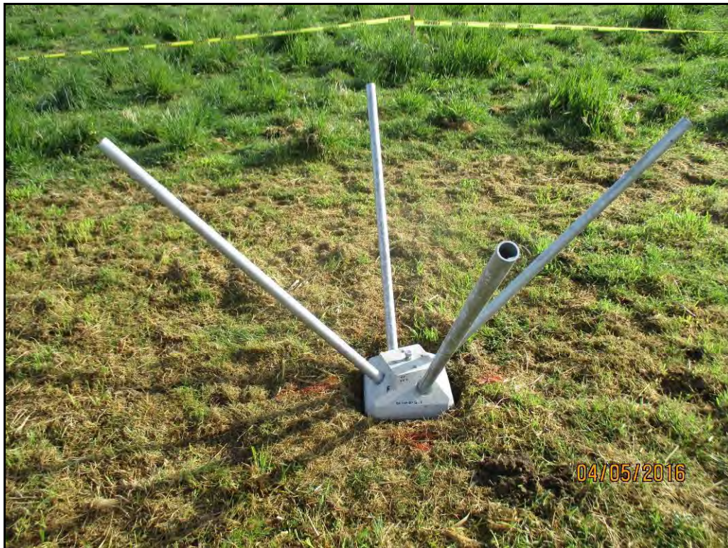
PHOTO 3: Typical concrete head seated and ready for bearing pin installation. Note caution tape in the background to ensure test site was not impacted by vehicular traffic surcharge loads.
