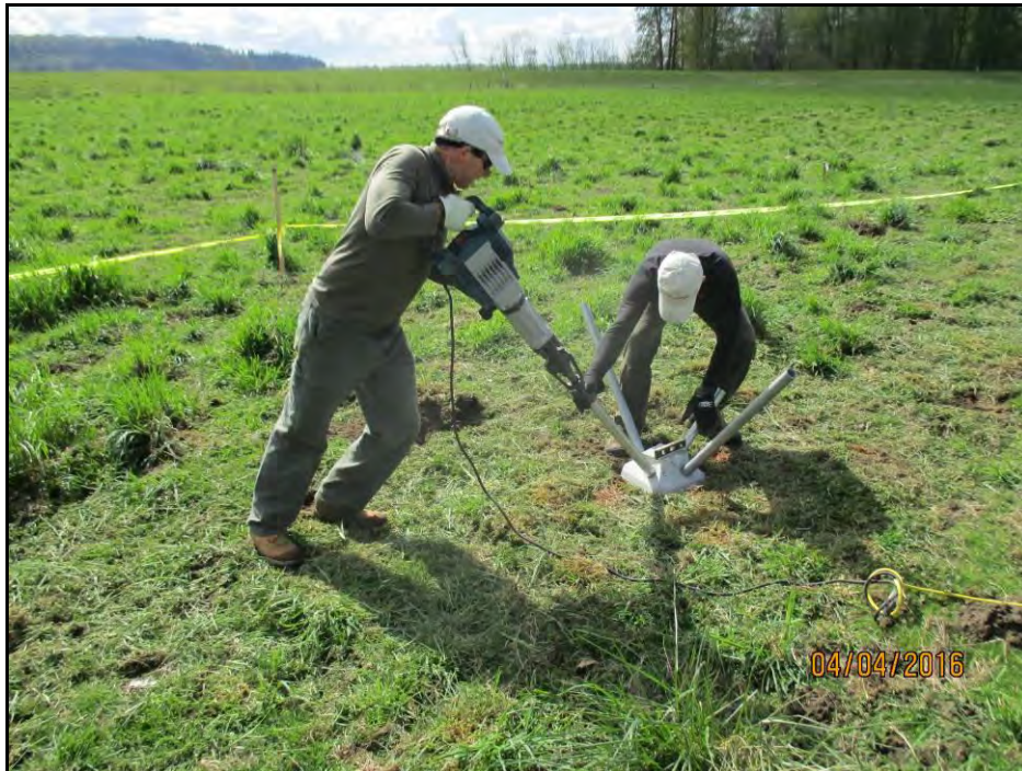
PHOTO 4: Typical driving of the steel bearing pins.
