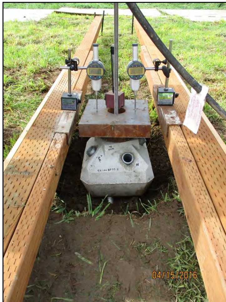
PHOTO 8: Typical uplift load test setup.
