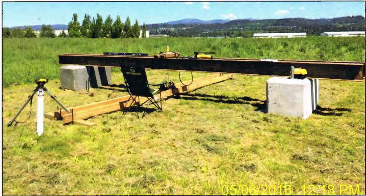
PHOTO 7: Typical uplift load test reaction frame setup.
