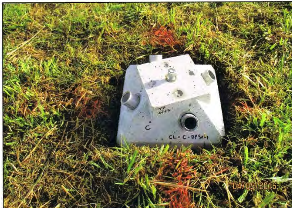
PHOTO 5: Typical Diamond Pier after the bearing pins were driven.
