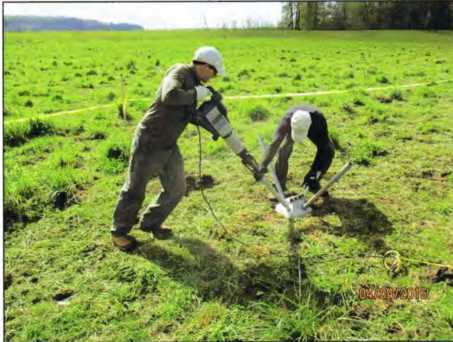
PHOTO 4: Typical driving of the steel bearing pins.
